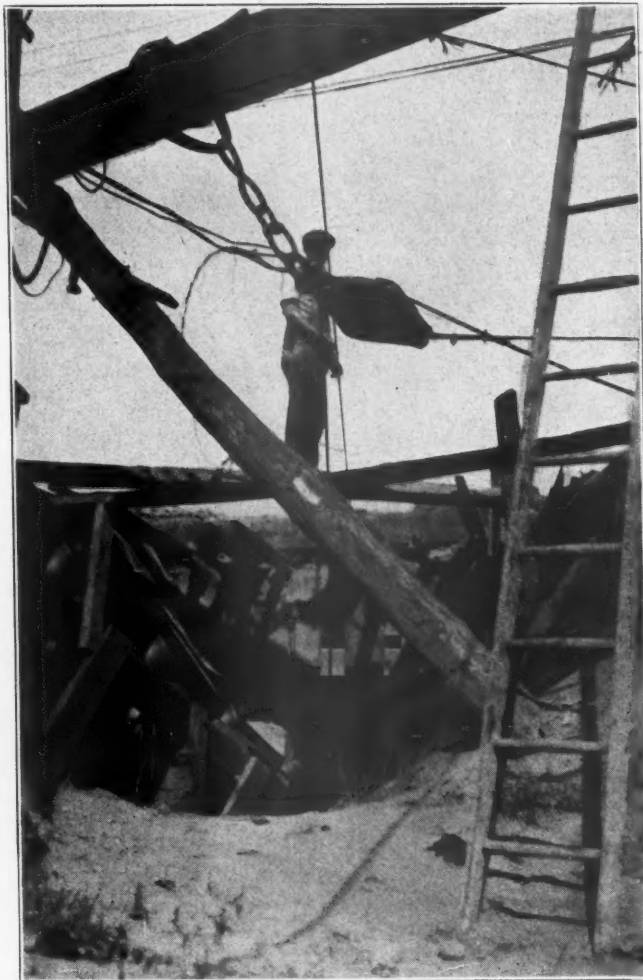
Lower End of Conveyor, Grizzly and Sheave for Drag Line. Cedar Grove
